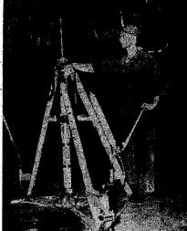
LOCAL PRODUCT JACK . . . Sgt. K. E. Kenny checks the locally fabricated nose wheel jack used by the 112th Tactical Reconnaissance Squadron before he begins a third intermediate inspection on a B-26 night photo recon stip.
